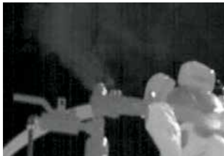
Thermal imaging with the GF306 can detect SF 6 leaks from plumbing or circuit breakers
