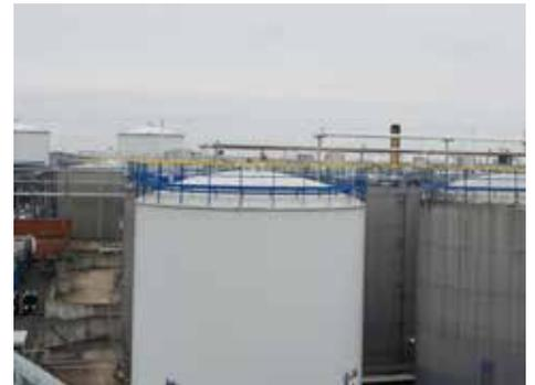
The ADPO site in the port of Antwerp has 276 tanks of varying sizes from 150m<sup>3</sup> up to 5.000m and stores more than 150 different liquids.
