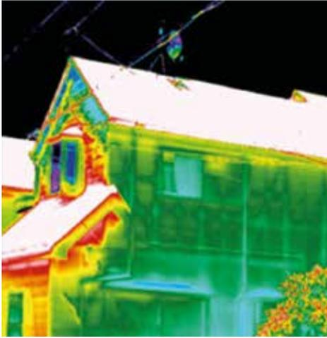
Figure 1 Thermal camera image
