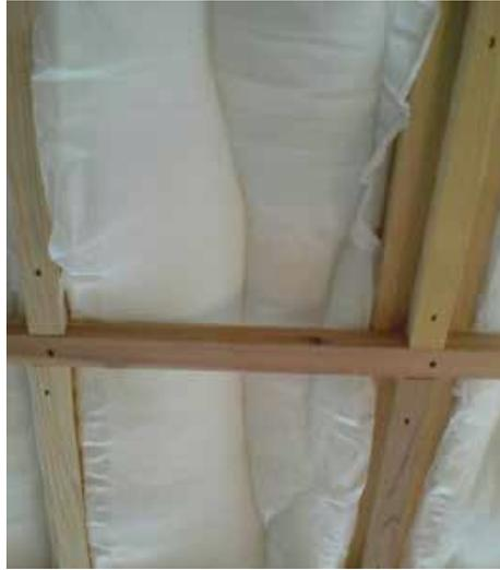
*Example of shoddy construction: There are spaces between insulation materials, resulting in an unwanted air current.*
