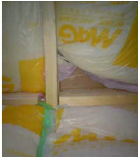
*Example of shoddy construction: the insulation left overturned after electrical work*
