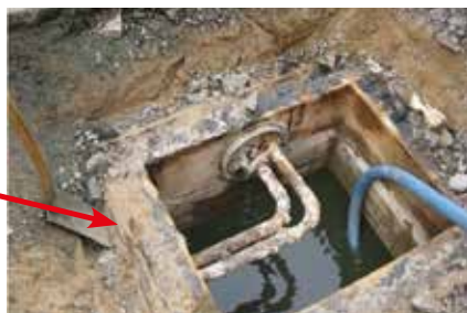
After seeing this leak in the report, the district heating company went there to investigate. It turned out to be a very large leak. Needless to say the company was very glad that this major leak was detected.
