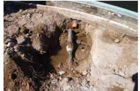
The repair workers were directed to open up the pavement where leaks were inspected, to find broken or cracked pipework, validating the results from the thermographic survey.
