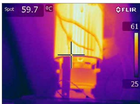
Looking for a hotspot on a lighting system
