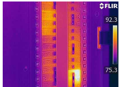
Overheating fuse in electrical panel
