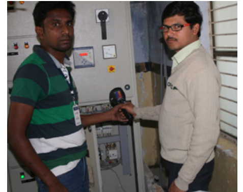
Nagesh,: "After performing a thermal audit with our FLIR i3 camera, we provide our customers with a report that certifies perfection in temperature and relative humidity maintenance."
