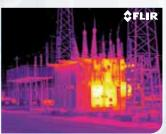
A transformer showing an excessive temperature.
