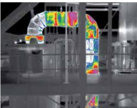
By showing temperature differences on the surface of the pipeline, hidden defects like leaks and missing insulation can be found.
