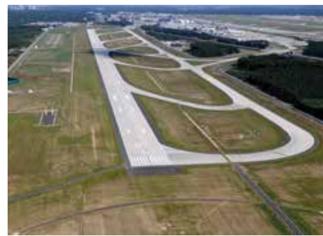
The new North/West runway (Photo: Fraport AG)
