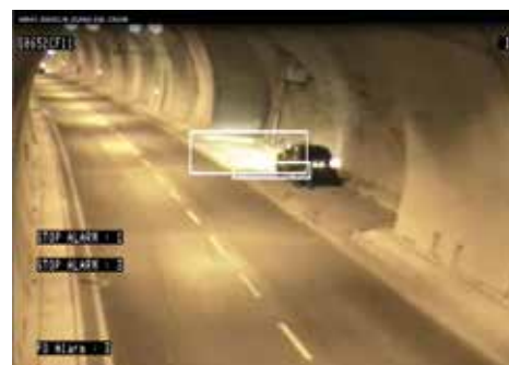
The Bolaman tunnel, the longest expressway tunnel in Turkey.
