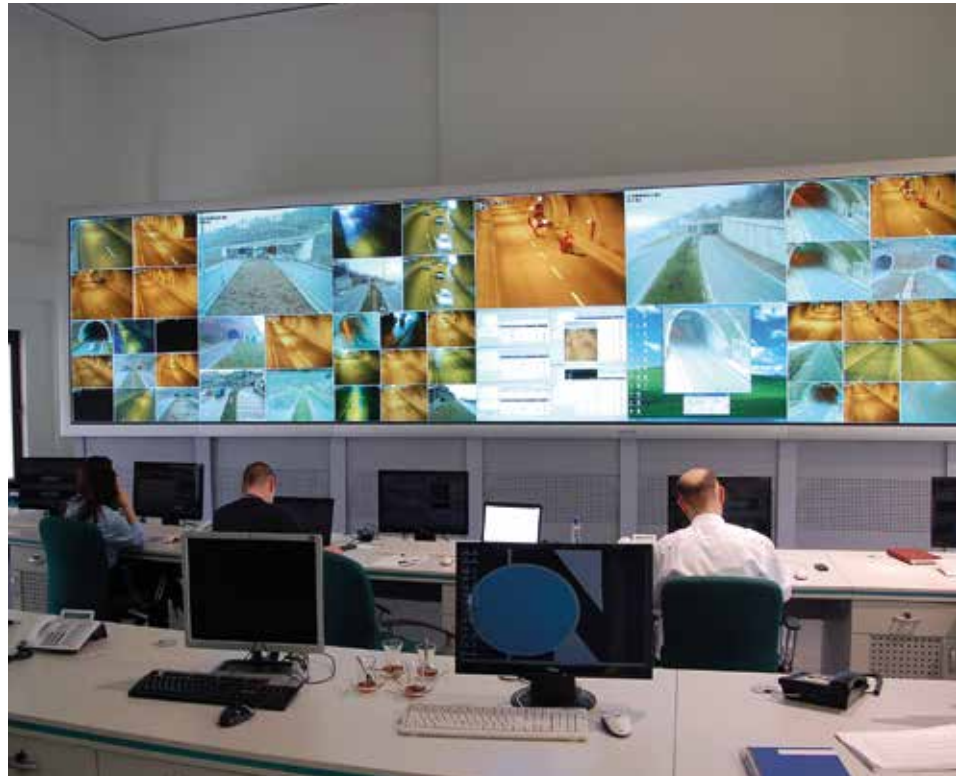
The traffic control centre in Trabzon, monitoring the tunnels on the Black Sea Motorway.
