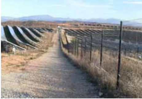
All along the perimeter a combination of fencing and thermal imaging cameras protects against intruders.
