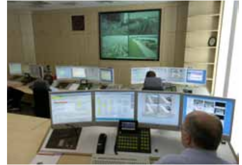
The BASF control room is the hub of the security network, where all footage from CCTV and thermal imaging cameras is analyzed.
