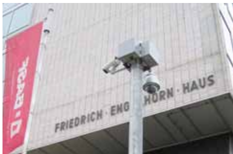
FLIR SR-Series thermal imaging cameras have been placed at strategic locations along the area's perimeter.
