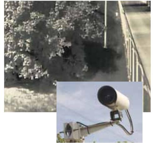
Branches moving in the wind caused many unwanted alarms in this location, so Krüger decided to replace the CCTV camera with a thermal imaging camera. Not one unwanted alarm has occurred since.
