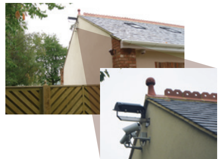
These two FLIR SR-313 thermal imaging cameras have adjacent fields of view, together they cover a large part of the surrounding fields.
