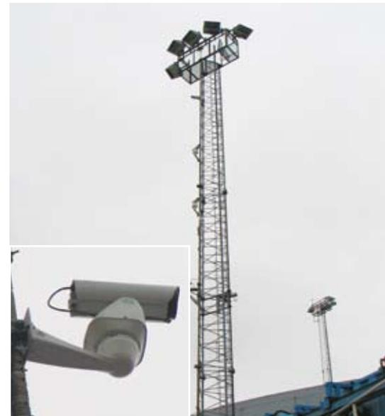
One of the FLIR Systems SR-100 thermal imaging cameras installed on a Pan/Tilt.
